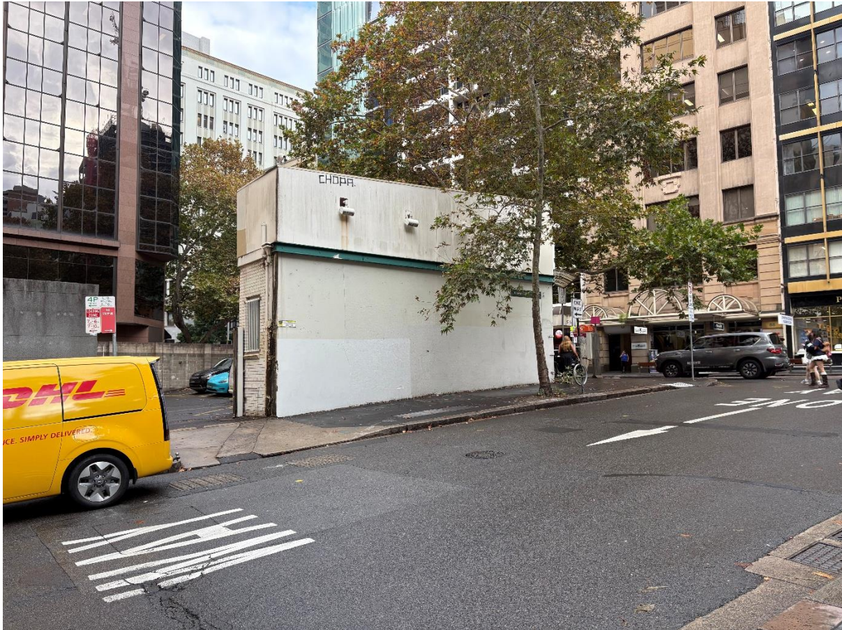
Figure 3: Site viewed from the northeast
