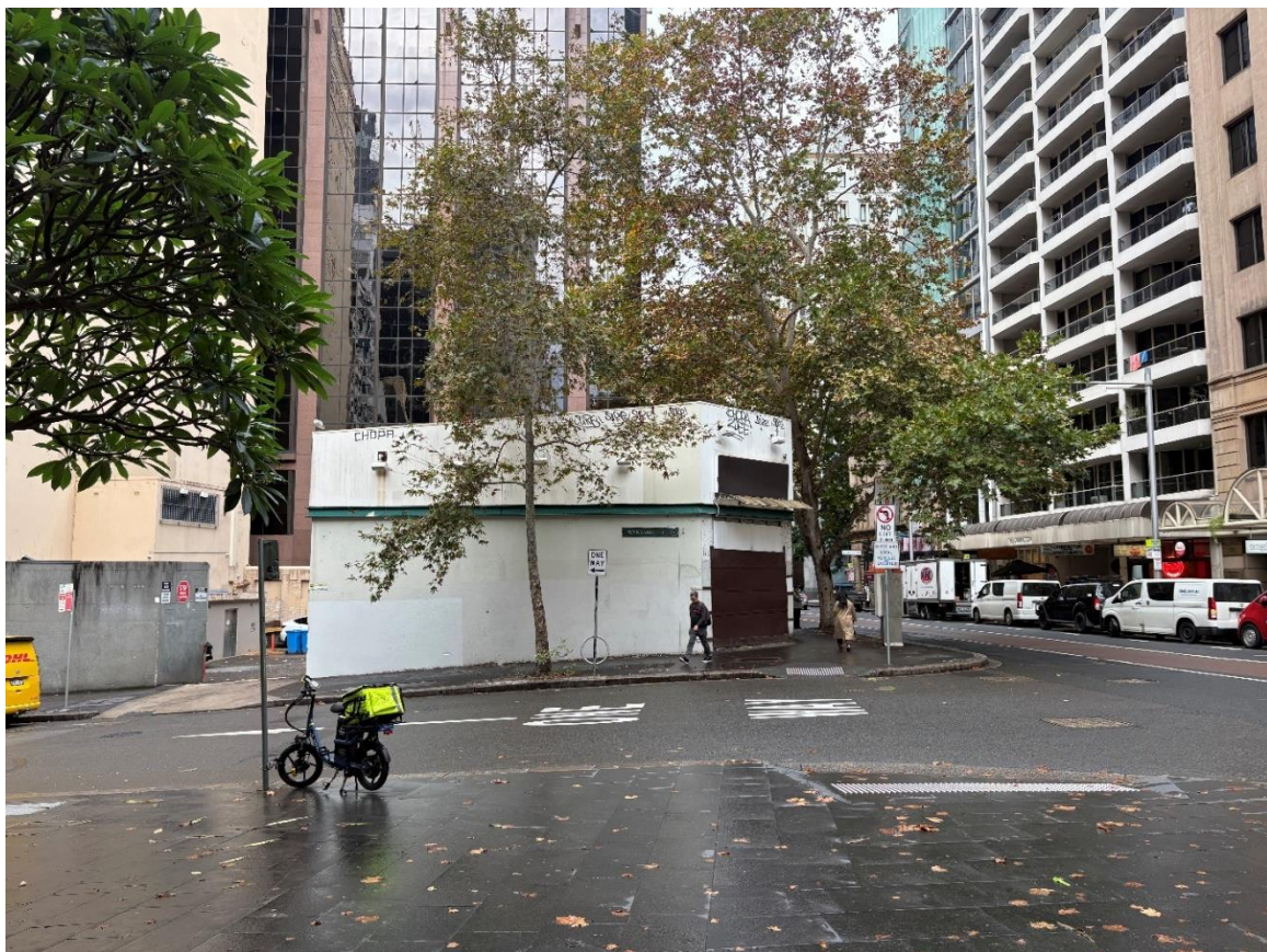
Figure 2: Site viewed from the north
